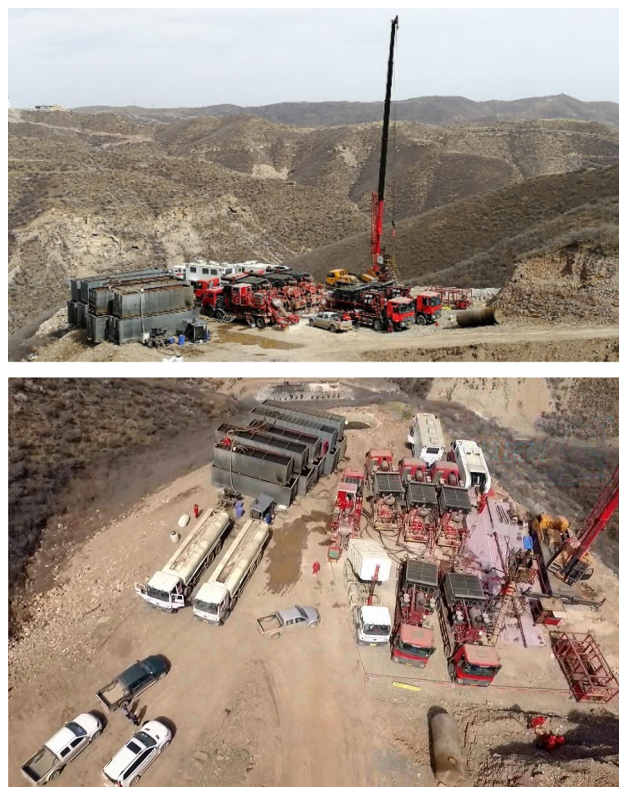
Fig. 9 Layout of construction site for ground fracturing (GF)
