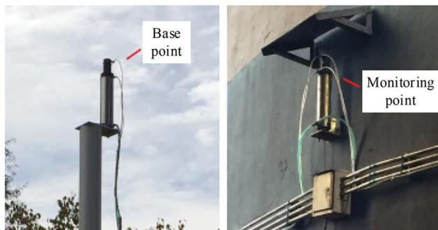
**Fig. 6** Installation of hydrostatic leveling system
