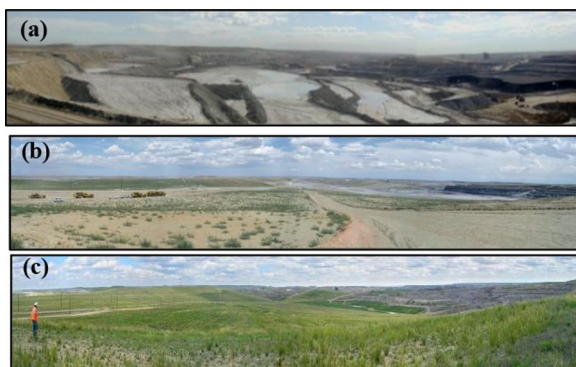
Fig. 2 Photos view east at the northern portion of West Pit collected from the same location a May 2005, b July 2006, area backfilled, c July 2010 area permanently seeded
