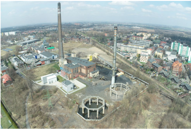
Fig. 4 Examples of technical infrastructure objects occurring on brownfield sites (Siemianowice Śląskie, Poland)
