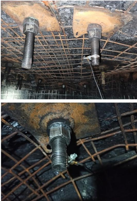
**Fig. 9** The investigated rock bolts in an underground opening in a working coal mine
