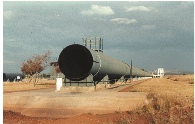
Fig. 2 Photograph of the 200 m test tunnel barrel and mouth
