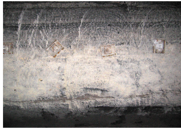
Fig. 4 Rib wall with bolt-plates visible on the surface
