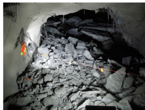
(b) A strain burst triggered by a fault-slip seismicity event (i.e., fault-slip burst event) in a metal mine at 1100 m of mining depth
