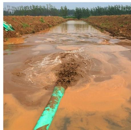
**Fig. 4** Filling and drainage of the water–sediment mixture in the reclamation strip. **a** Filling; **b** Drainage
