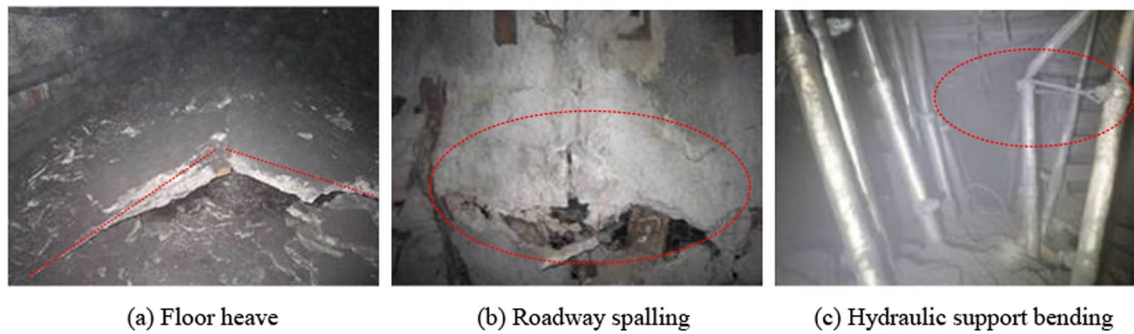
Fig. 2 Overstress failures in mine workings in the Datong mining area (Yu et al. 2014; Mou 2021)
