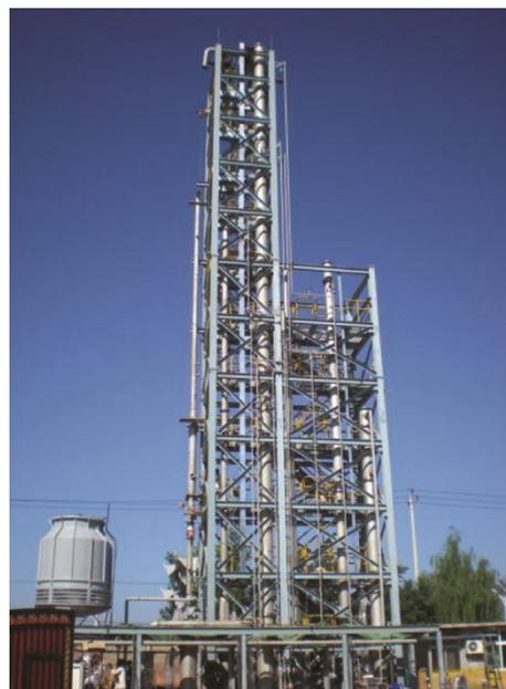
**Fig. 7** CO<sub>2</sub> capture verification plant for natural gas flue gas located in Beijing
