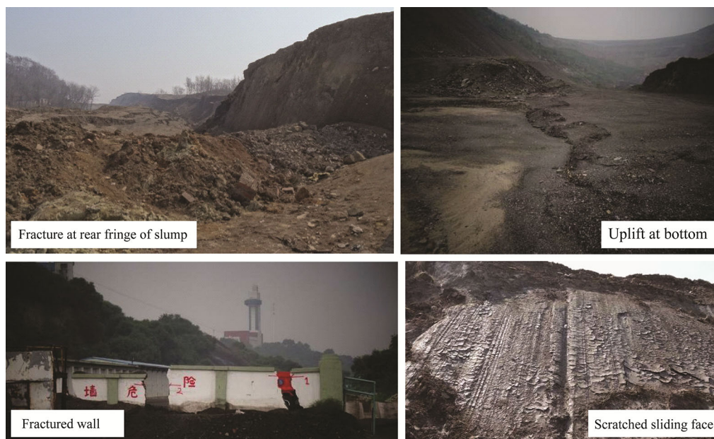
Fig. 4 Landslide-induced surface phenomena
