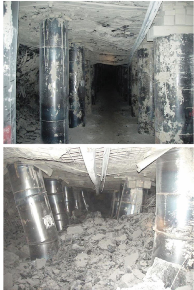
Fig. 2 Effect of a coal burst on a longwall tailgate
