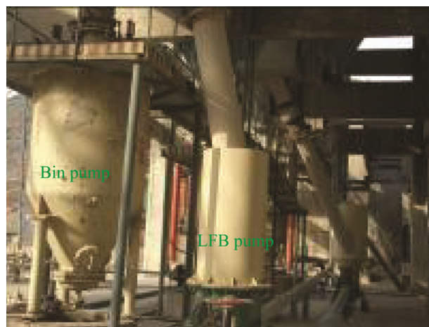
Fig. 13 The application of the material sealing pump
