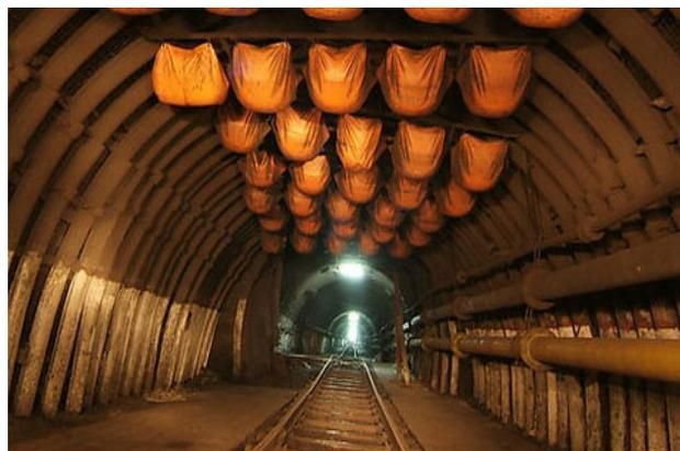
Fig. 2 Water barriers in Chinese underground coal mines
